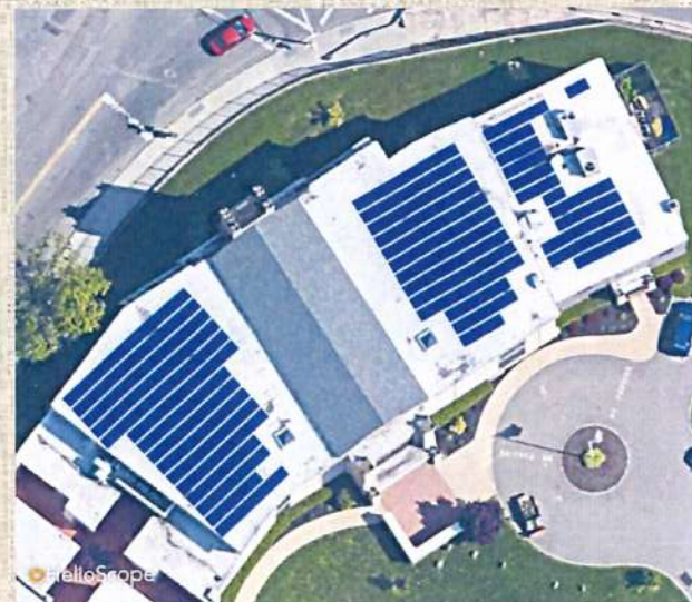
Solar Panels over St. Joseph's Mausoleum
